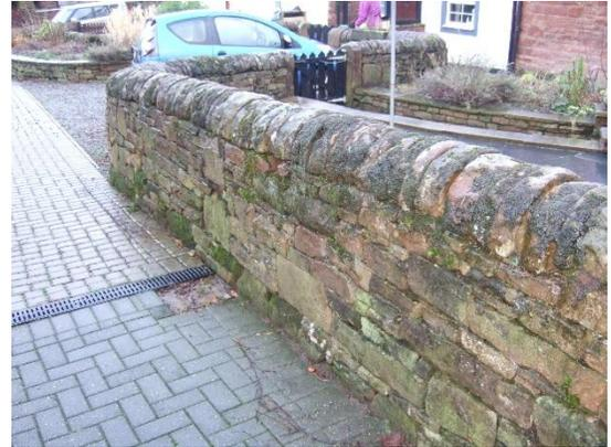
Figure 27 Sandstone wall with rounded capping
