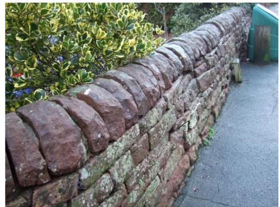
Figure 28 Sandstone wall with rounded capping
