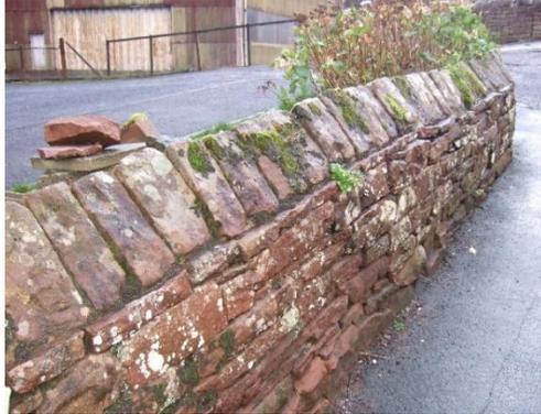
Figure 24 Sandstone wall with triangular capping
