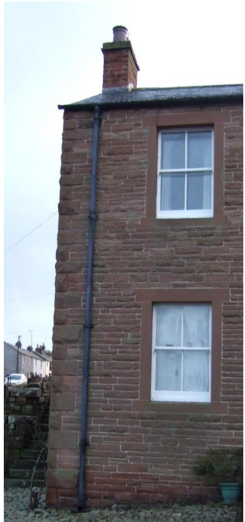
Figure 15 Typical decorative style from the village with emphasised quoins at the wall corner, simple junction with the eaves and flush fitting sandstone window surrounds. The walls are rough-dressed sandstone ashlars
