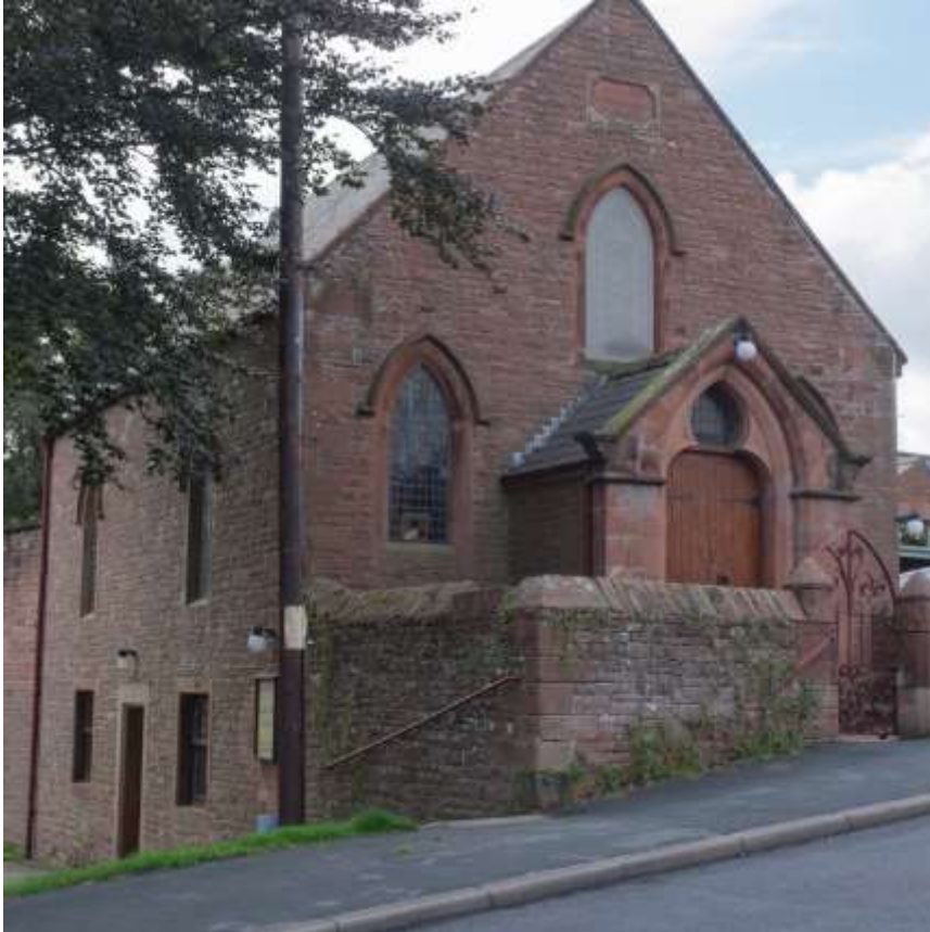
Fig 17 Former Methodist Chapel, potential location for café
