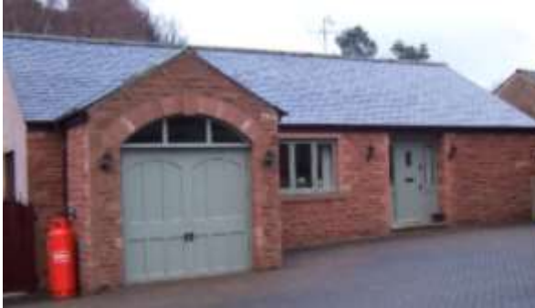
Figure 17 Modern house reflecting the architectural detailing seen in older houses. Emphasised quoins at wall corners and forming the arch above the garage and dressed window surrounds with lintels and sills formed from single pieces of sandstone
