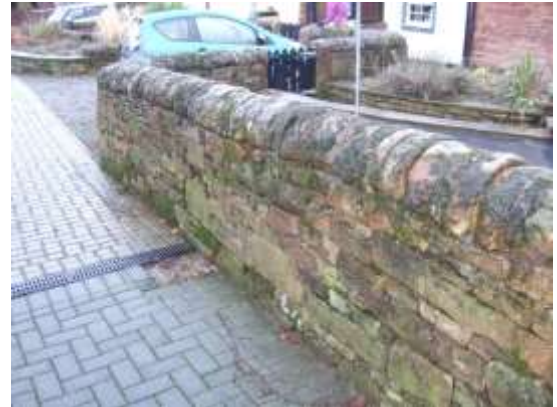
Figure 27 Sandstone wall with rounded capping
