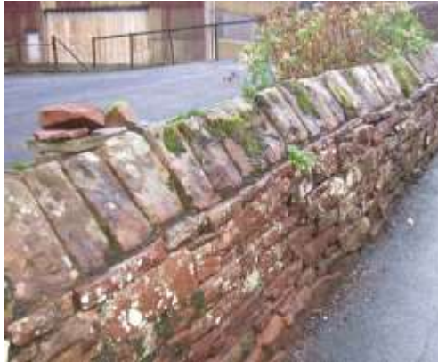
Figure 24 Sandstone wall with triangular capping
