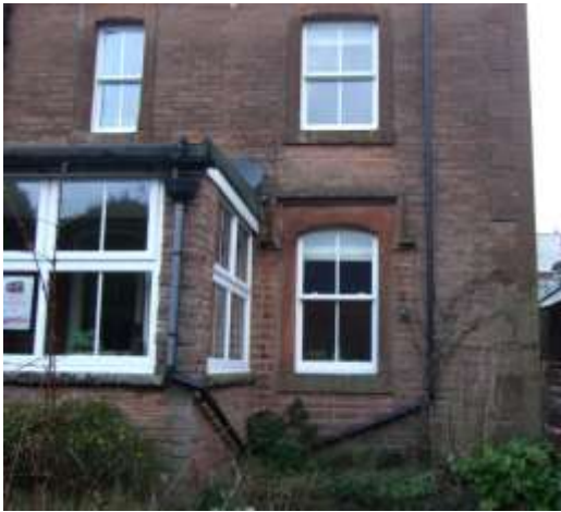
Figure 18 Another typical village house of rough-dressed sandstone ashlars and dressed ashlars to emphasise the corners of the main house. The front extension is not of the same quality
