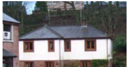
Figure 4 Modern house with slate roof
