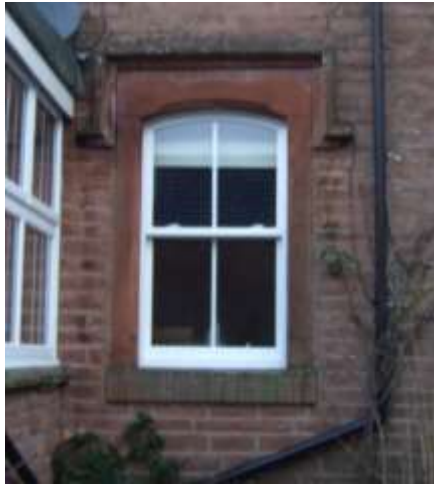
Figure 20 Ornate window with moulded hood
