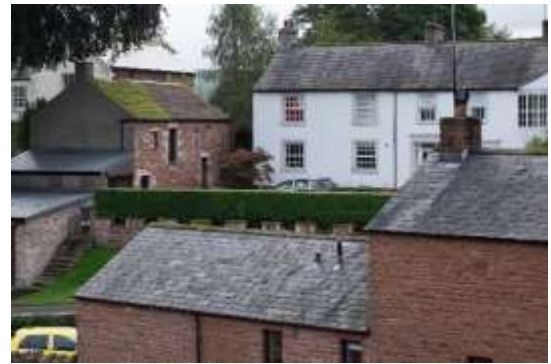
Figure 29 A variety of roofs: slate in foreground and background, with sandstone slabs on building to left with modern profile sheeting on lean-to
