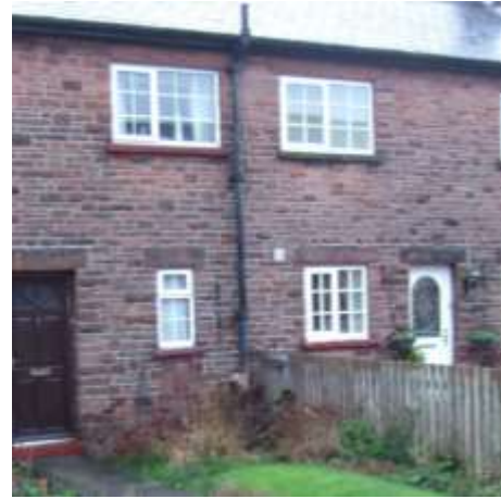
Figure 23 Fairly modern houses with side-hung casements. The windows have a sandstone lintel above, a sandstone sill and undressed sides. The windows are mix of top- and side-hung casements
