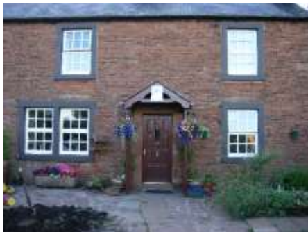
Figure 22 Characteristic sandstone window surrounds that have been painted. The windows are six-over-six modern casement windows
