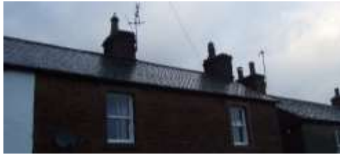
Figure 32 A pair of traditional houses with slate roofs
