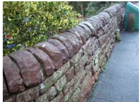
Figure 28 Sandstone wall with rounded capping
