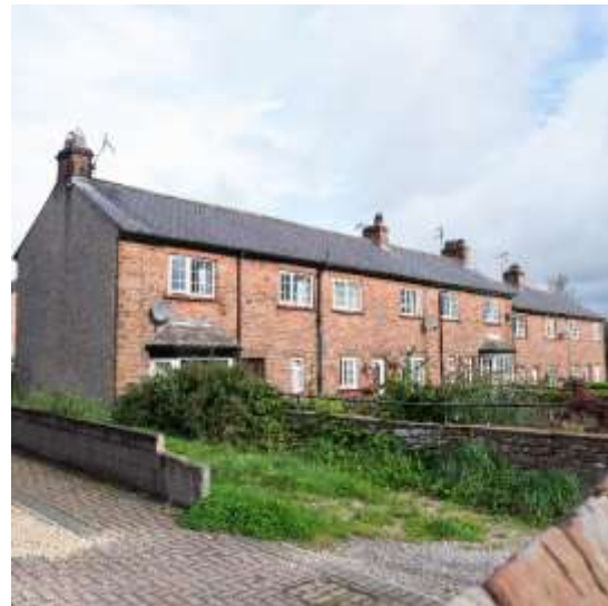
Figure 37 Terrace of recent houses opposite the Village Hall with sandstone facades and rendered gables
