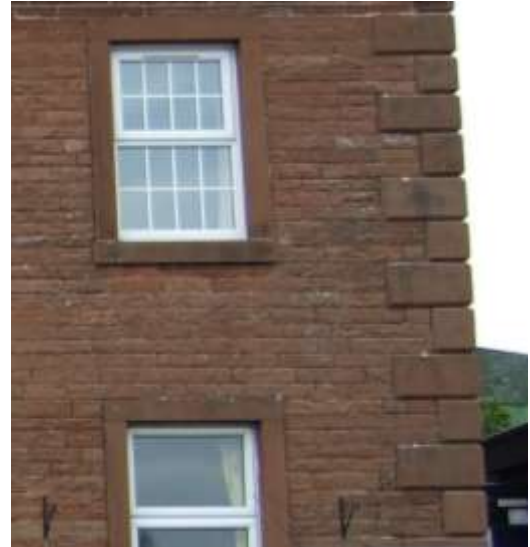
Figure 10 V-jointed sandstone quoins
