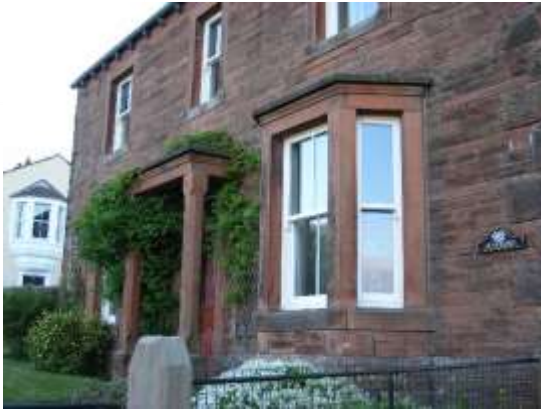
Figure 12 This house has a number of decorative flourishes. Note the projecting bay window, the pillared porch, the emphasised quoins at the corners of the house, and the dentillation at the eaves. there is also an angular sandstone gate-post in the foreground
