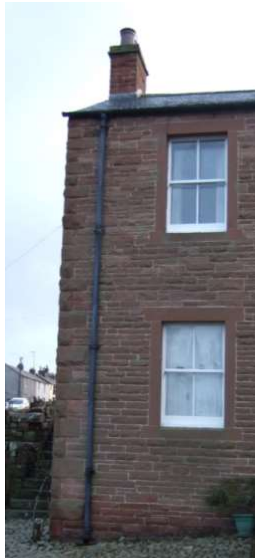
Figure 15 Typical decorative style from the village with emphasised quoins at the wall corner, simple junction
